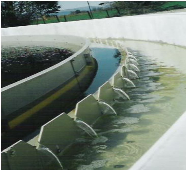
Scum boards, Weir plates and Baffle boxes manufactured to specification with durable ISOTHALIC GELCOAT and completely sealed edges to prevent frosting and cracking.
